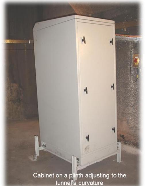
Cabinet on a plinth adjusting to the tunnel's curvature
